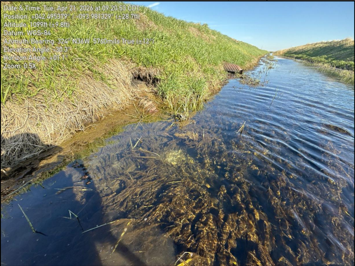
Broken and submerged tile outlets.
