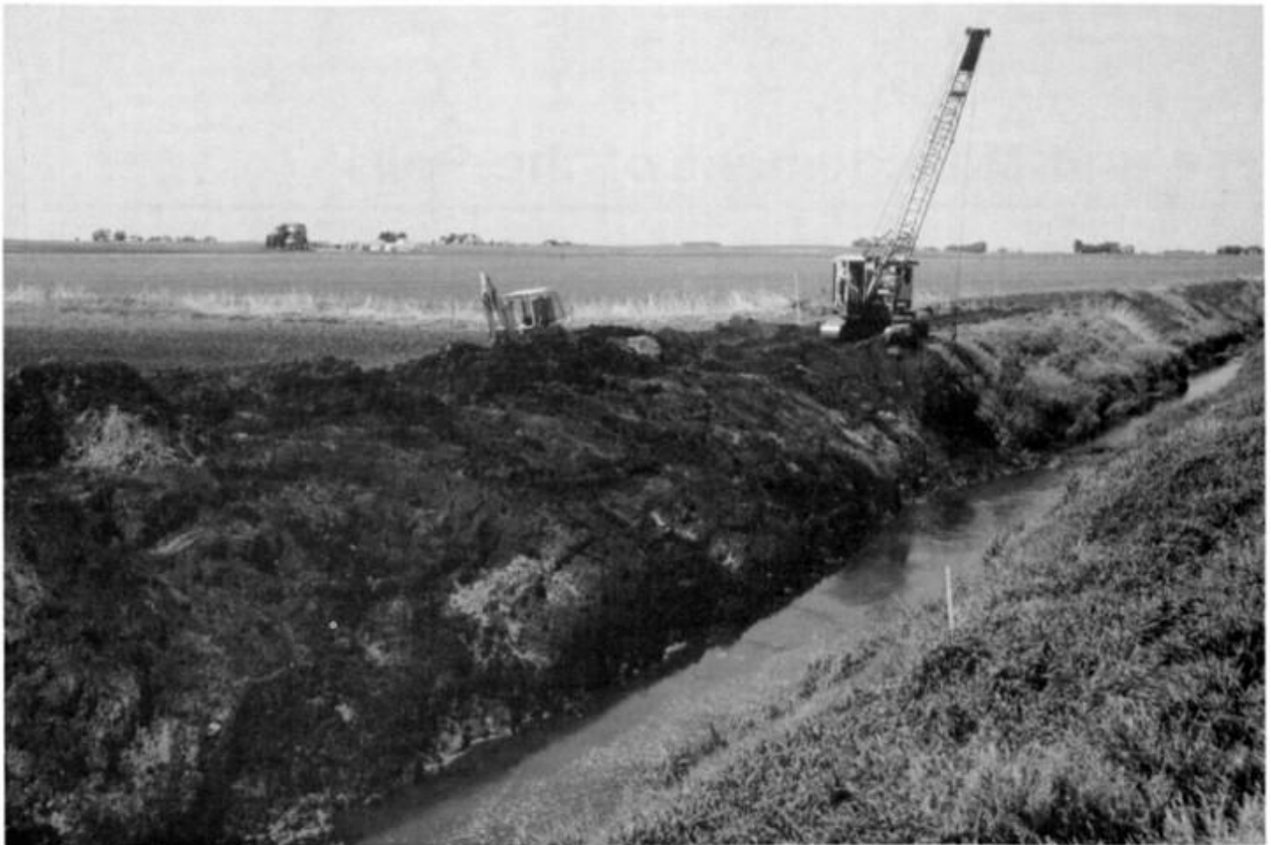
Figure 12. A drainage ditch through an area of Canisteo silty clay loam, 0 to 2 percent slopes. Drainage ditches provide outlets for subsurface tile.
