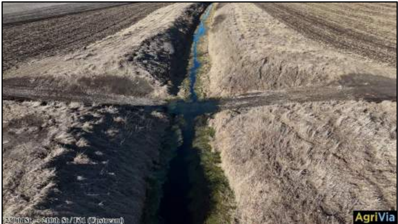
Ford crossing to be lowered to match design flowline.
