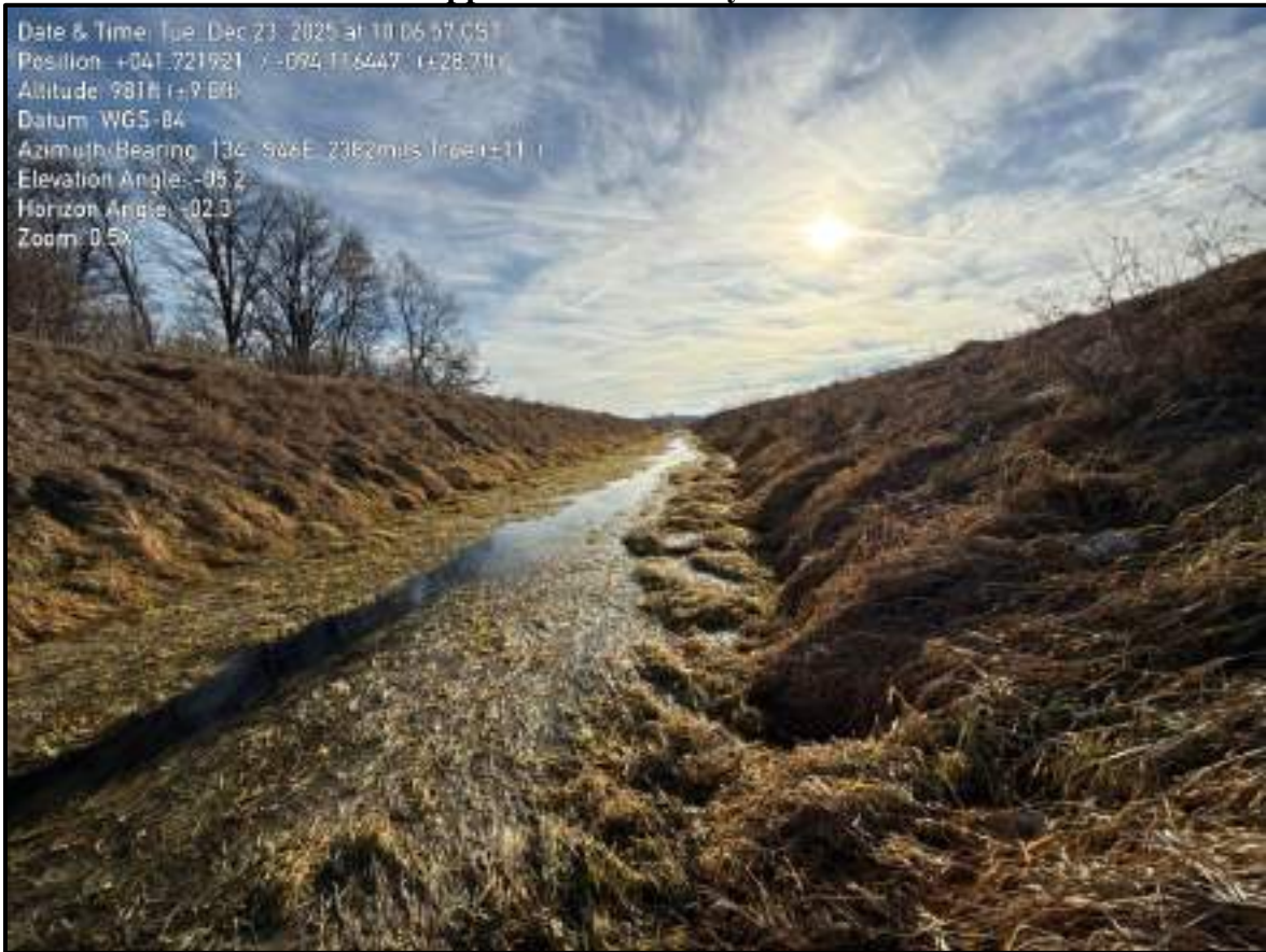
Open Ditch in Section 16
