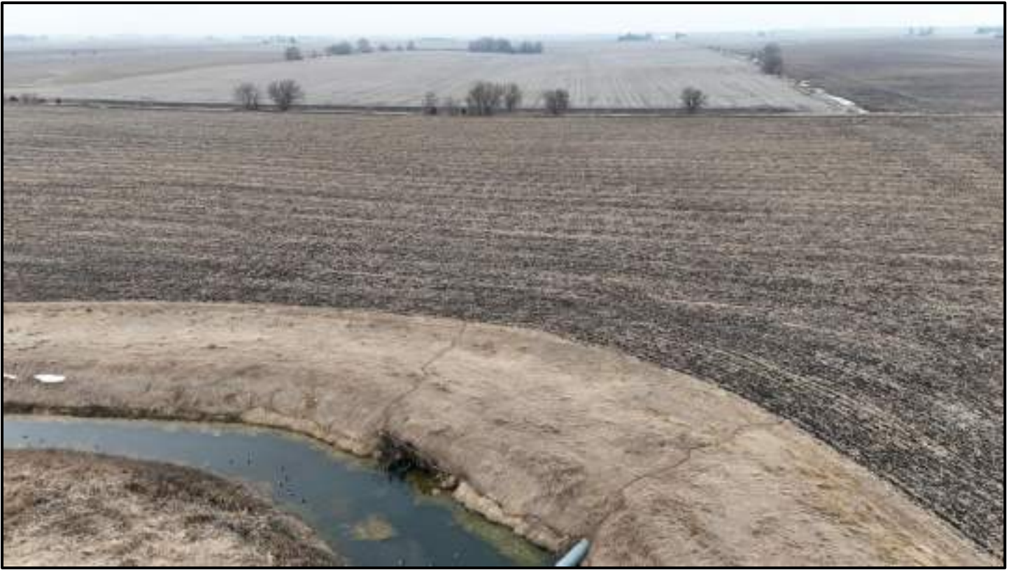
Open Ditch and Branch No. 1 Bulkhead
