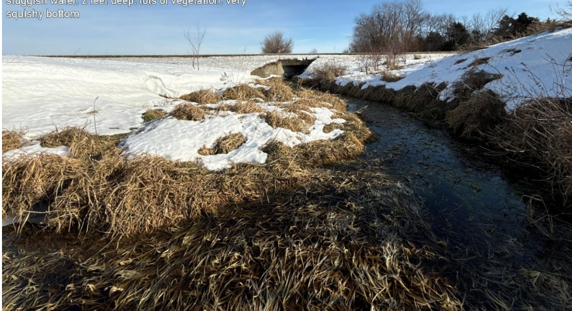
3- Downstream Ditch- Culvert
